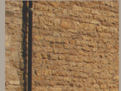
An example of a local limestone rubble walling
