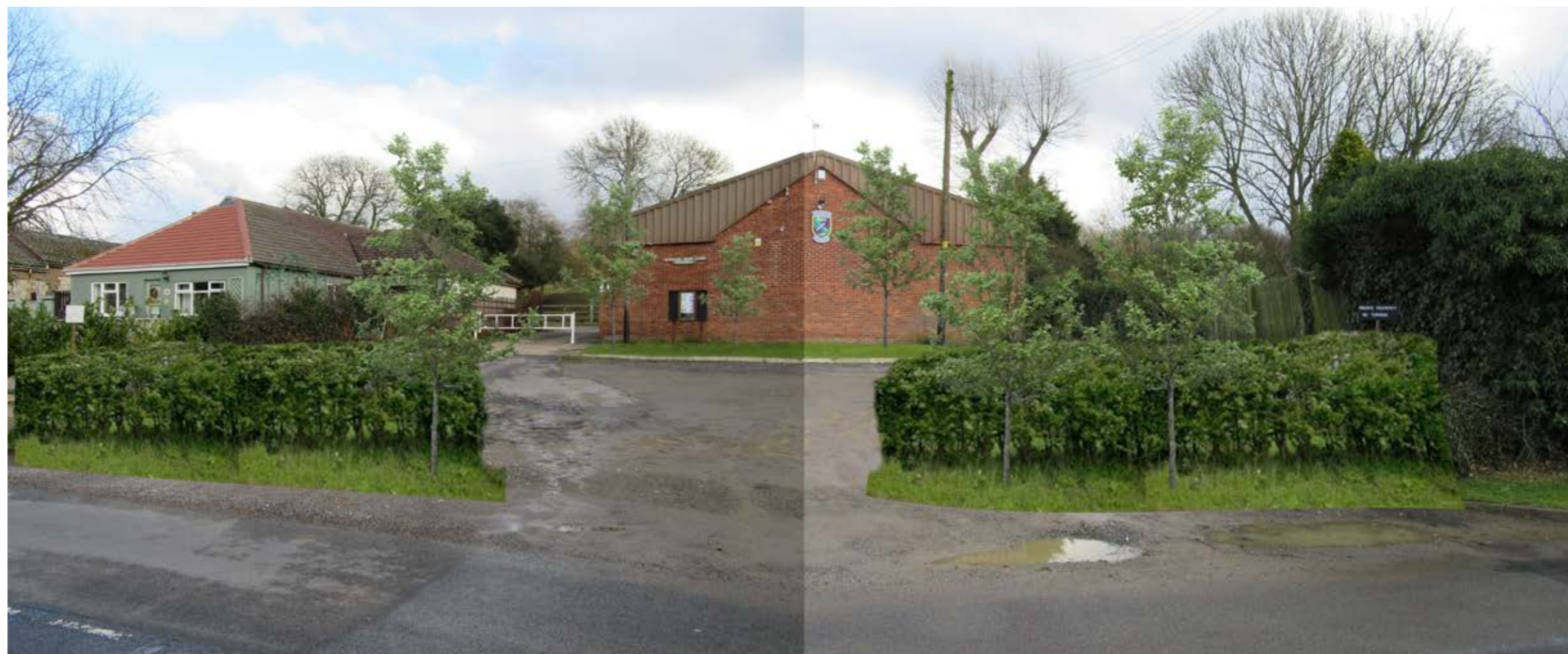
Fig 203: The above photoshopped image demonstrates how simple retrospective planting schemes can improve the appearance of a building and improve its relationship with the wider village context.
