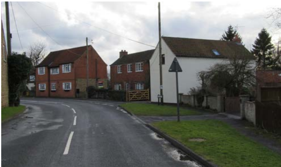
Fig 163: Large detached dwellings, with simple pitched roof forms and red brick or white rendered façades terminate the view looking south towards where Weldon Road meets Bunkers Hill.
