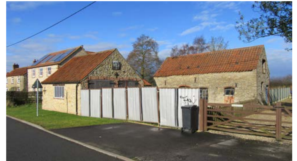
Fig 77: The former smithy buildings represent some of the most unique and charming vernacular structures at Brook Street, however, the full splendour of their form cannot be appreciated due to the presence of a rather blunt and unsympathetic boundary treatment.
