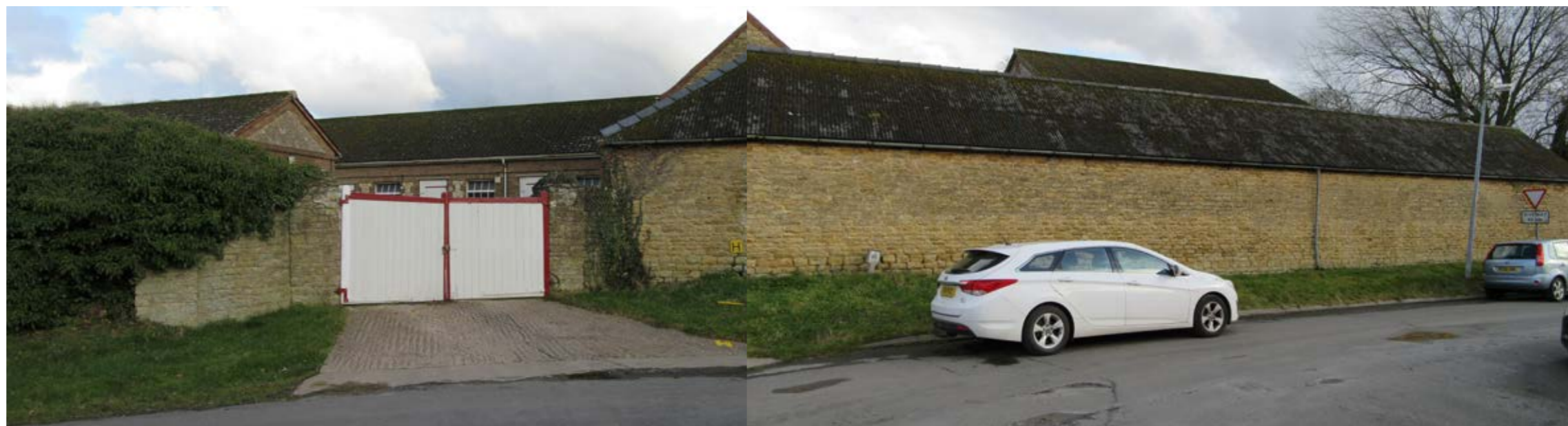
Fig 107-109: The buildings of Stud Farm and Poplar House form a distinct and important grouping along the eastern side of Dawnhill Lane.
