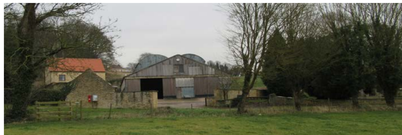
Fig 275: Built with functionality in mind, the large sheds at Church Farm are rather rudimentary in their form and appearance, though their downbeat colouration makes them a generally subservient presence along this part of Common Lane. More unfortunate is the loss of the escarpment trees that has previously provided these buildings with a soft wooded backdrop
