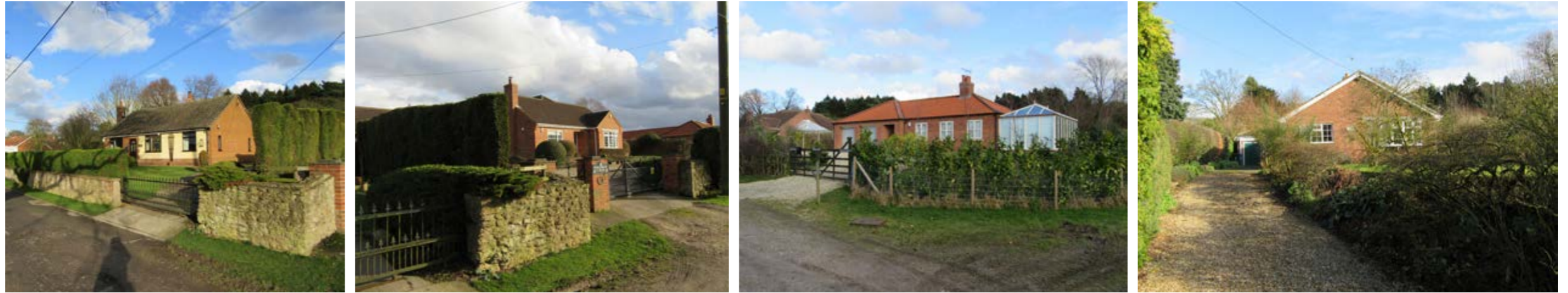
Fig 185-188: Development along the south-eastern side of Weldon Road largely comprises detached bungalows of differing architectural languages, but which are tied together through similar positioning in relation to the roadside (slightly set-back behind shallow front gardens), the use of red brick as their primary construction material, the progression of hedgerows and stone walling along property boundaries, and finally, the constant presence of the rising profile of the cliff landscape as their backdrop.
