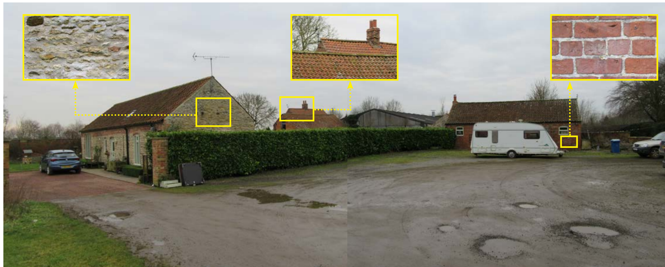
Fig 248: To the immediate south of Hall Farm lies a large surface car parking area edged by formal garden hedgerows and a couple of modest single storey buildings of similar linear form with pitched roofs. Finished in local stone and with a pantile roof is the Old Stables building, now a dwelling, whilst further west is a similarly scaled, red brick finished property, now used as a furniture-making workshop. Set to the rear of these buildings, and largely screened in views from the car park, are several agricultural buildings associated with Hall Farm, including several old red brick and pantile roofed sheds whose rooftops emerge as interesting features in views beyond the band of hedgerows.
