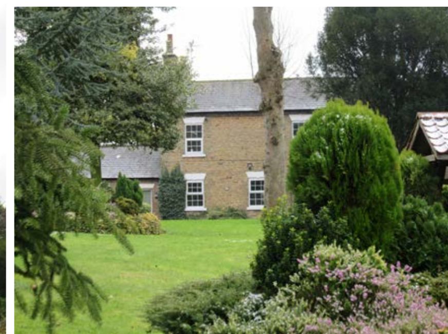
Fig 294 and 295: Partial views of Hermitage Farm can be gained from Church Lane through the beautifully landscaped grounds it lies within. From this viewpoint is possible gain an appreciation its built fabric and aesthetic qualities.
