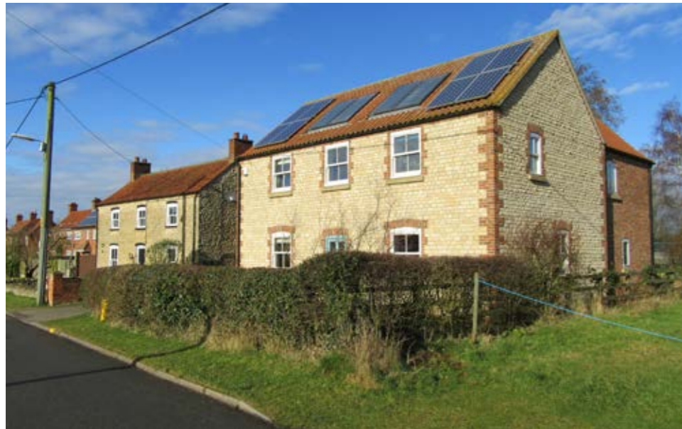
Fig 75: No.17a is recent addition to the northern side of Brook Street, which replicates the vernacular aesthetic of the more historic coursed stone properties that neighbour it.
