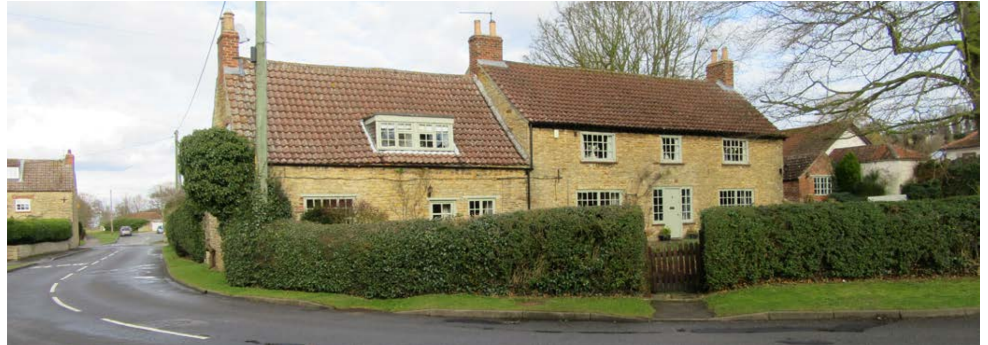
Fig 164: The 17th century Spring Cottage is one of the highlights of the Bunker's Hill gateway into Hemswell. This striking dwelling has an extensive yet well-proportioned coursed stone facade, accommodating both small pane casement windows and also horizontal sliding sash windows.
