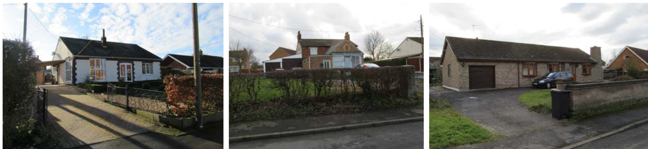
Fig 79 -81: The southern side of Brook Street has a particularly mixed character, with each dwelling progressing its own unique aesthetic, and paying little regard to the village's established architectural languages and vernacular forms. Even the former village store building (centre), which represents the most historic property along this row, has been altered beyond recognition, and in a particularly ad-hoc manner, with numerous additions to the building's front and side.
