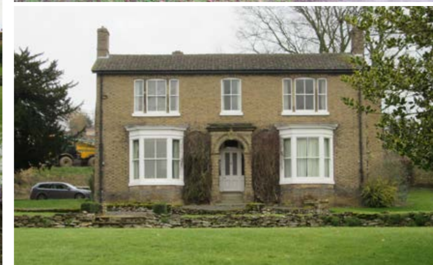
Fig 269 and 270: Church Farm is one Harpswell's most iconic and handsome residential buildings, and its locally distinct stone walling is crucial streetscape element along the central stretch of Common Lane.
