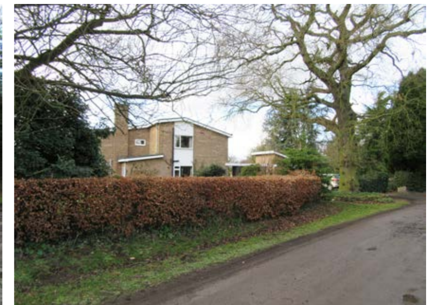
Fig 235: Bellwood, despite its more modern architectural leanings, still integrates into its rural setting due to its setback positioning from the road, mature gardens and planted boundary.
