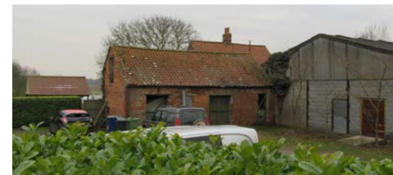
Fig 250: Several of the sheds at Hall Farm were actually constructed from the bricks of the arched garden wall that formed part of the ornamental gardens of Harpswell Hall.
